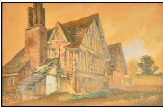
Left: Selly Manor in the late 19 th century showing its timber frame and tall brick chimneys. The tiled roof and some of the brickwork were later additions. Right: A panel of wattle and daub.
