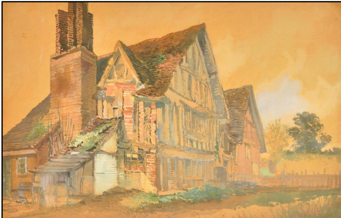
Above: Selly Manor in the late 19 th century showing its timber frame and tall brick chimneys. The tiled roof and some of the brickwork were later additions. Right: A panel of wattle and daub.
