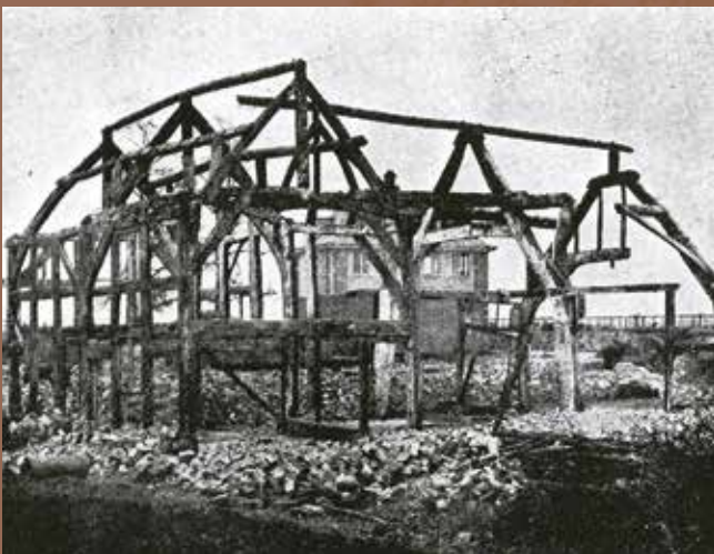
Minworth Greaves in its original location.
