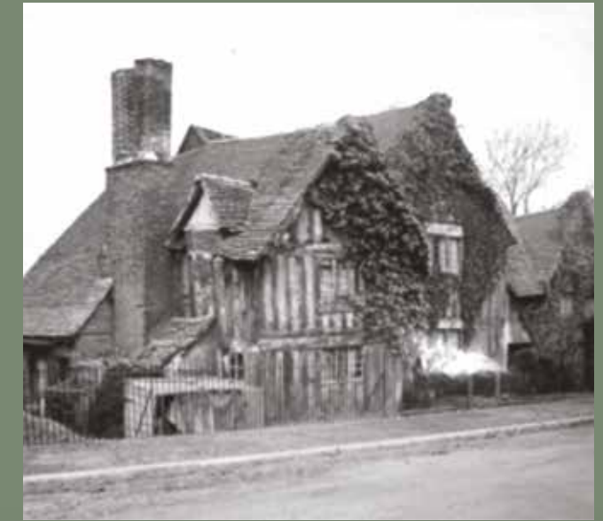
Image taken in 1904 in its original location on Bournbrook Road.
