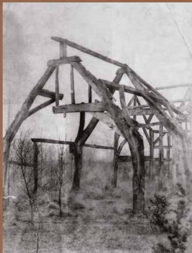
Minworth Greaves at the time it was purchased by Harvey, the bent oak timber known as crucks are clearly visible.
